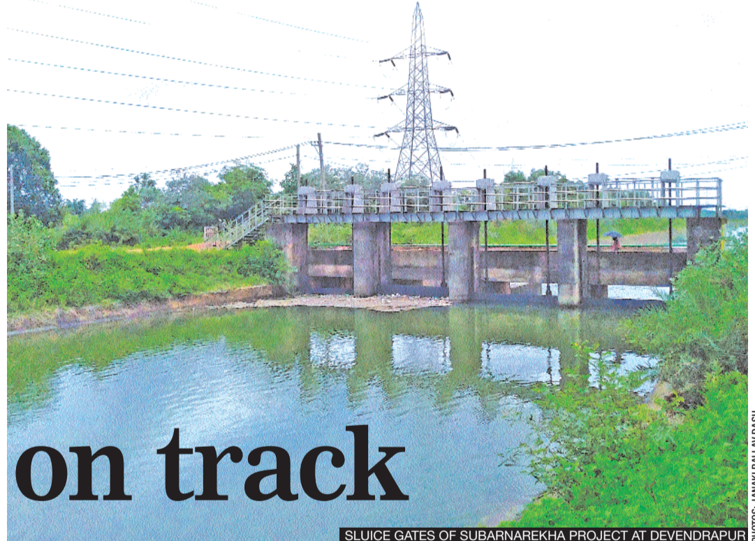
SLUICE GATES OF SUBARNAREKHA PROJECT AT DEVENDRAPUR
